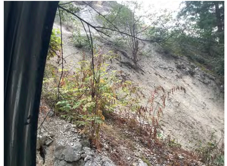
Left bank downstream fill slope
